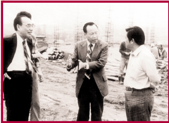
Groundbreaking: Taiwan's seminal Hsinchu Park took shape under Irving Ho, M.S. '57, Ph.D. '61 (center).
